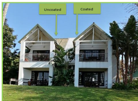
Figure 2: View of adjoining application and reference bungalow
